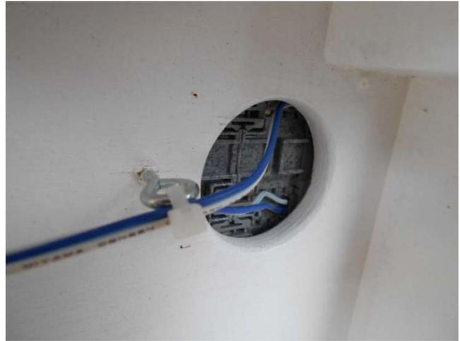
This photograph shows the Cup Hooks and Screw Eye under the module.
